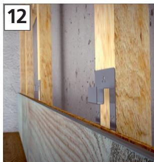
After this, further panels can be inserted in **Plane 3** or Row 3 can be continued using a panel in **Plane 1**. All panels in **Plane 1** in Row 3 are again to be secured using a 3D profile claw. For this, a profile claw must be mounted into each counter batten. The profile claws are to be arranged in such a way that the opened side of the claw body is facing downwards [12].
